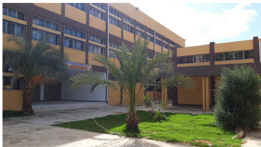
SIRTE (LIBYA) Al-Yarmouk school after rehabilitation. Photo: ©UNDP Libya
