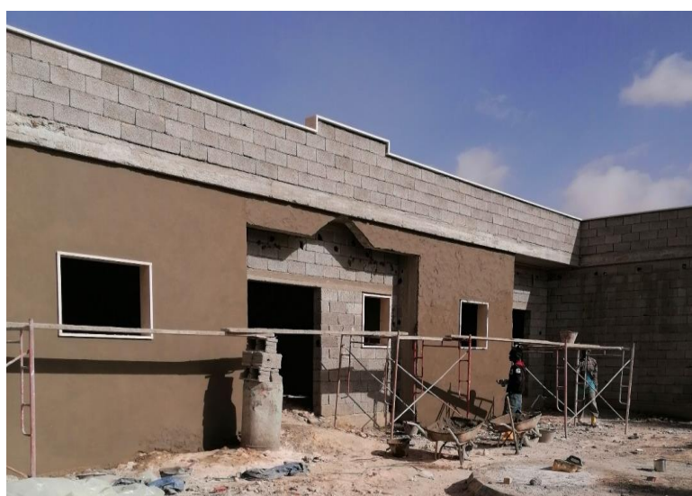
BANI WALID (LIBYA) Ongoing works to establish isolation facility in Bani Walid General Hospital. Photo: ©UNDP Libya
